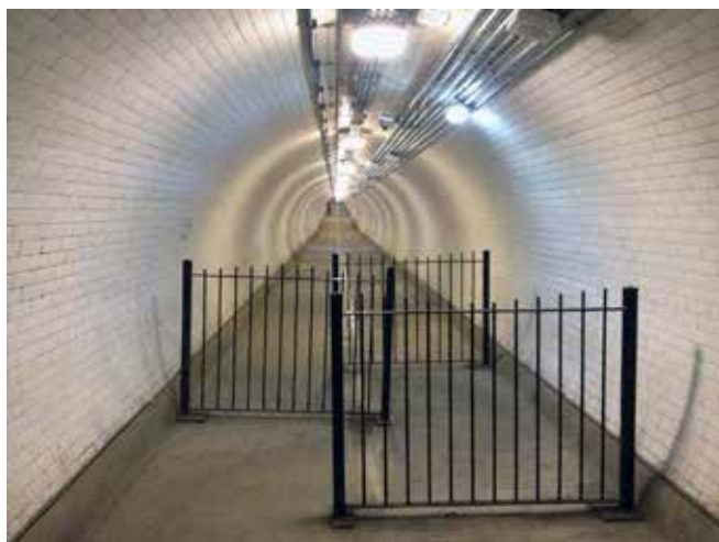
After refurbishment the tunnel is looking clean and bright much as it did on the opening day. Photo Andy Hebden
